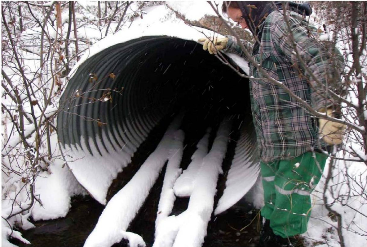
Figure 4-4 Equalization culvert between Mink Arm and South McMahon Lake
