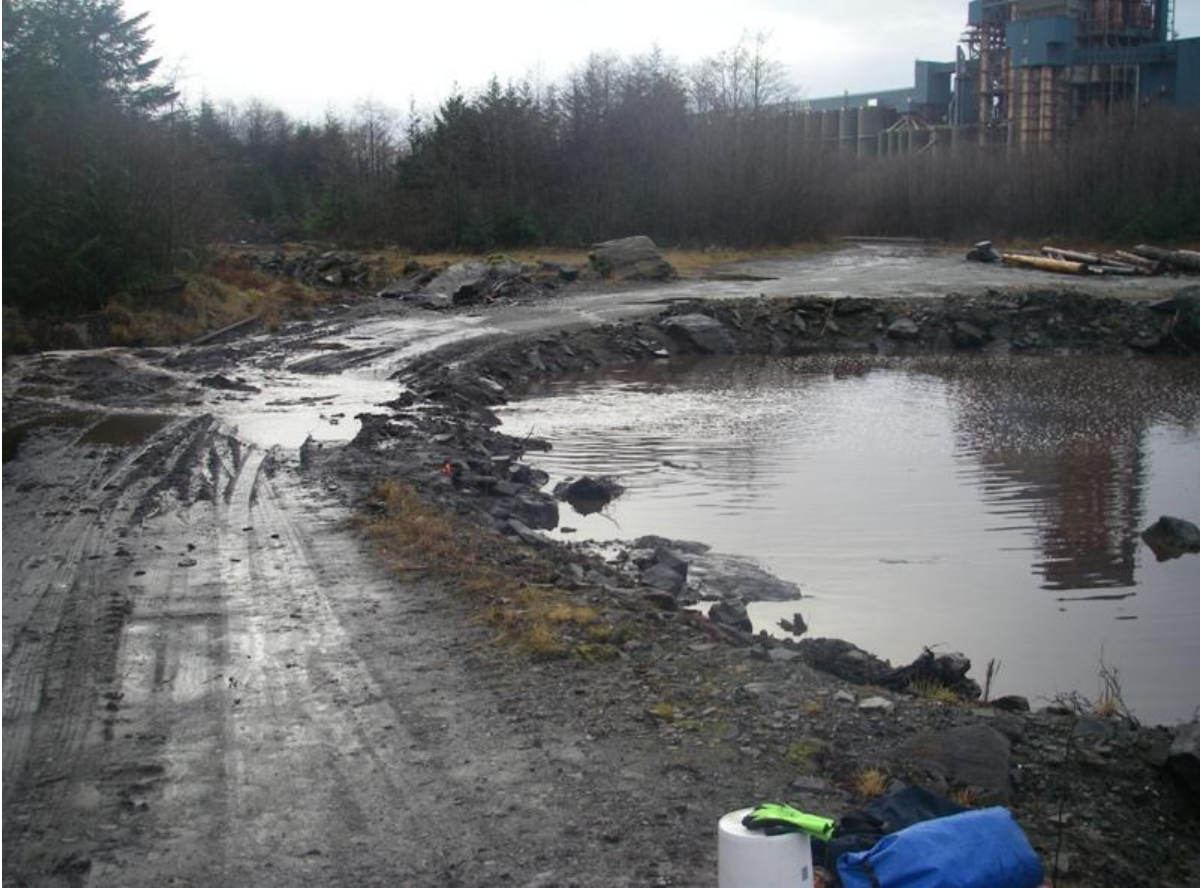
Photo 4: Berm on south end of tidal pond that lacks culvert to stream. Runoff from Ridley Island Log Sort can be seen flowing across the road from left to right in foreground.
