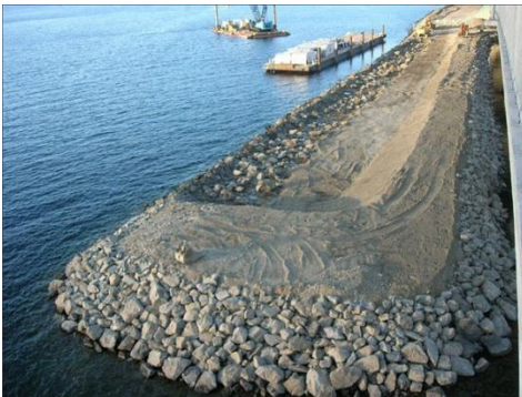
Example of causeway construction With riprap protection
