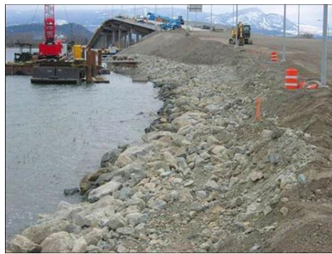
Example of an earthfill causeway and bridge
