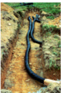
Figure 3.8 Photograph of trench and drainage lines
