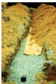
Figure 3.9 Photograph of the filling in of a drainage trench
