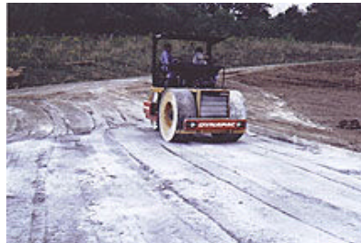
Figure 3.4 Photograph of the compaction of an impermeable pad during construction
