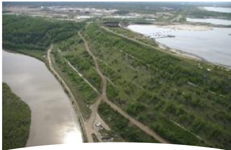
THE TAR ISLAND DYKE IS NOTORIOUS FOR LEAKING CONTAMINATED WATER DIRECTLY INTO THE ATHABASCA, BUT ALL TAILINGS PONDS LEAK.
