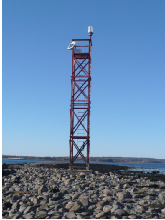
Figure 1b: Steel tower.
