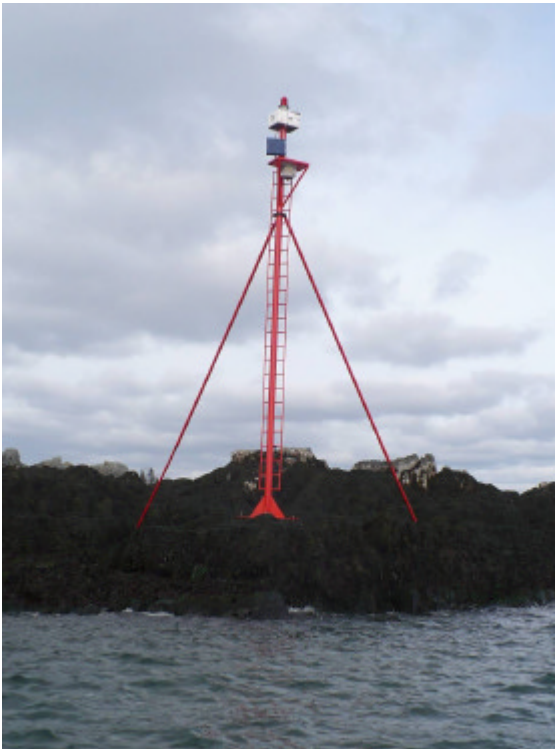
Figure 1c: Spindle structure with braces.
