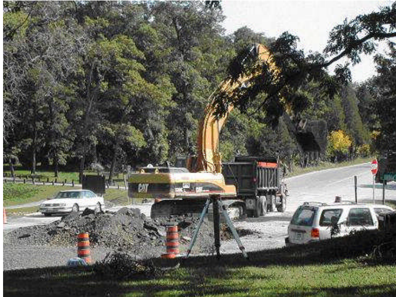
Photo 7: Intersection improvements (Manitoba SHIP)
