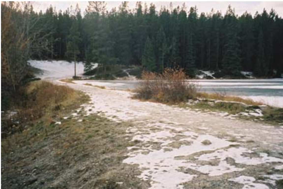
Photo 2. Berm at east end of Johnson Lake, November, 2002. Berm prevents flows to the east and resulting in dry streambeds at M54L Poles 249-248, 253-252 and 259-258.
